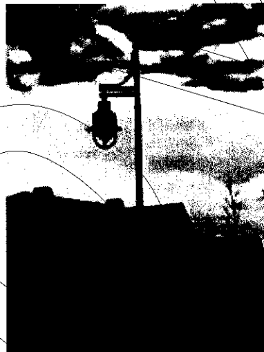
Figure 3-13: Typical Street Lighting
